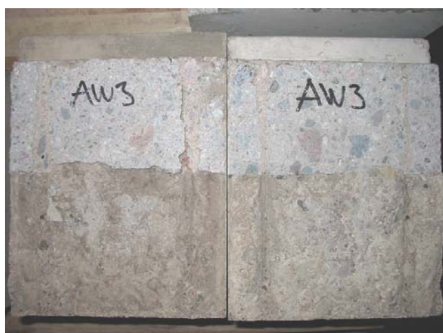
Figure 15 The joint in test W-A3 after testing.
